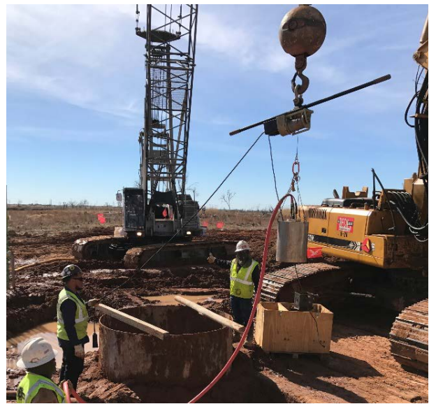
b) Mini-SID lowered into the drilled hole
